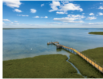
Beach & Bay Access with 7 Beach Walkovers and Elevated Boardwalk Over Drum Bay Nature Preserve
